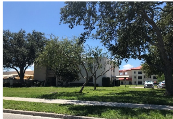
Photo 5: Existing After School Care Facility (“P3”)
